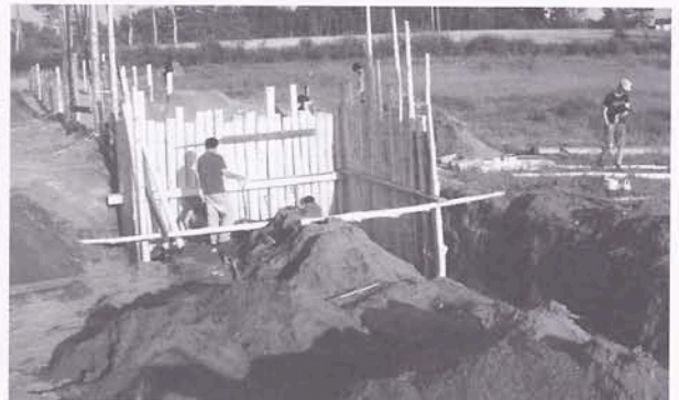
Retaining wall under construction (2008).
