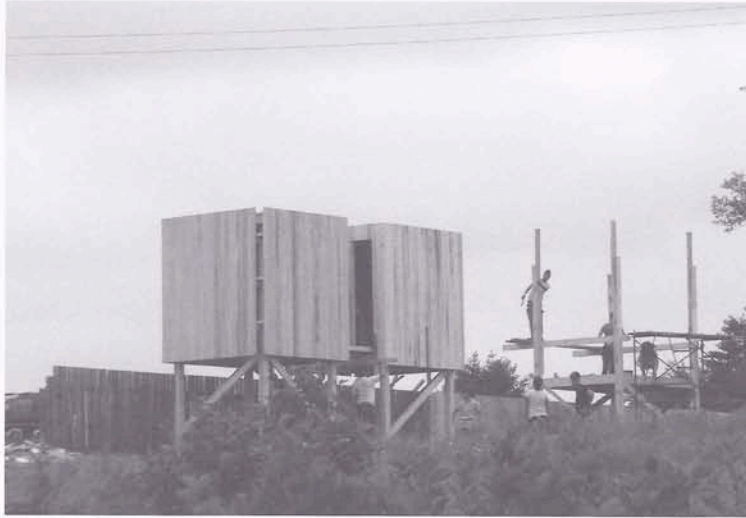
View of accommodation nearing completion (2010).
