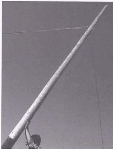
Raising a mast as screen support.
