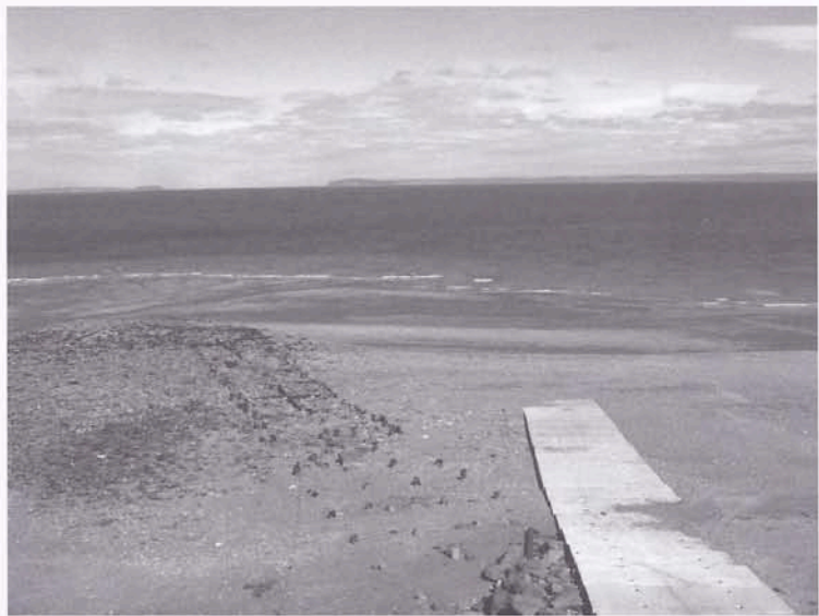
view of cribwork for historic wharf and new concrete slip.
